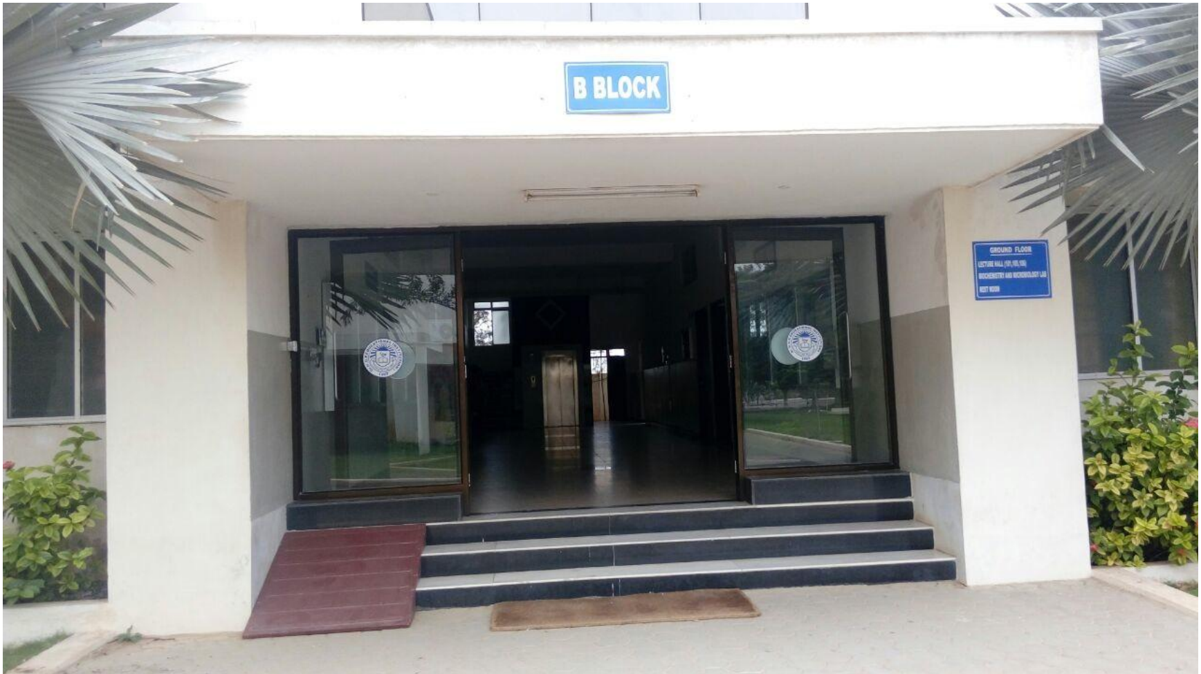
Ramp - B Block
